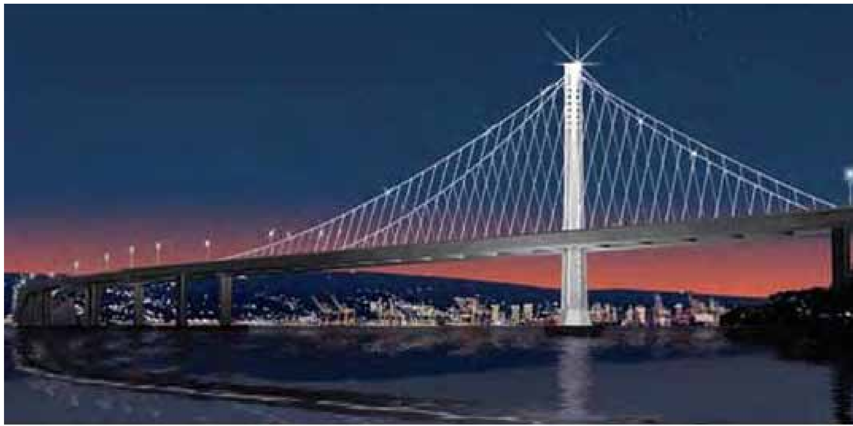
The Bridge is meant to glow at night, an orchestrated event
