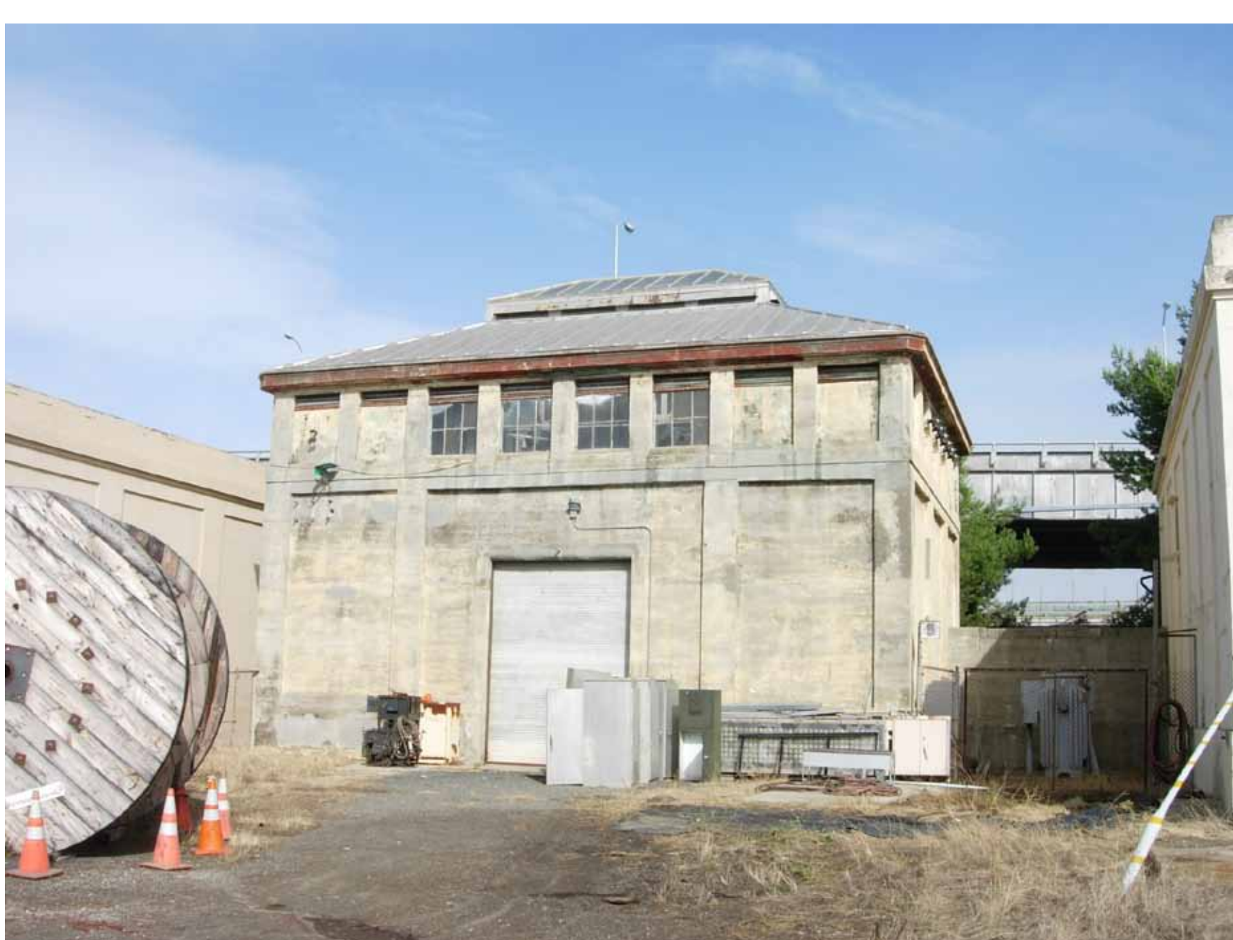
Key Pier Substation
