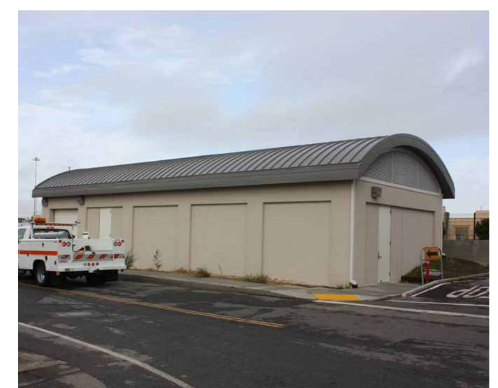
Caltrans Maintenance Building
