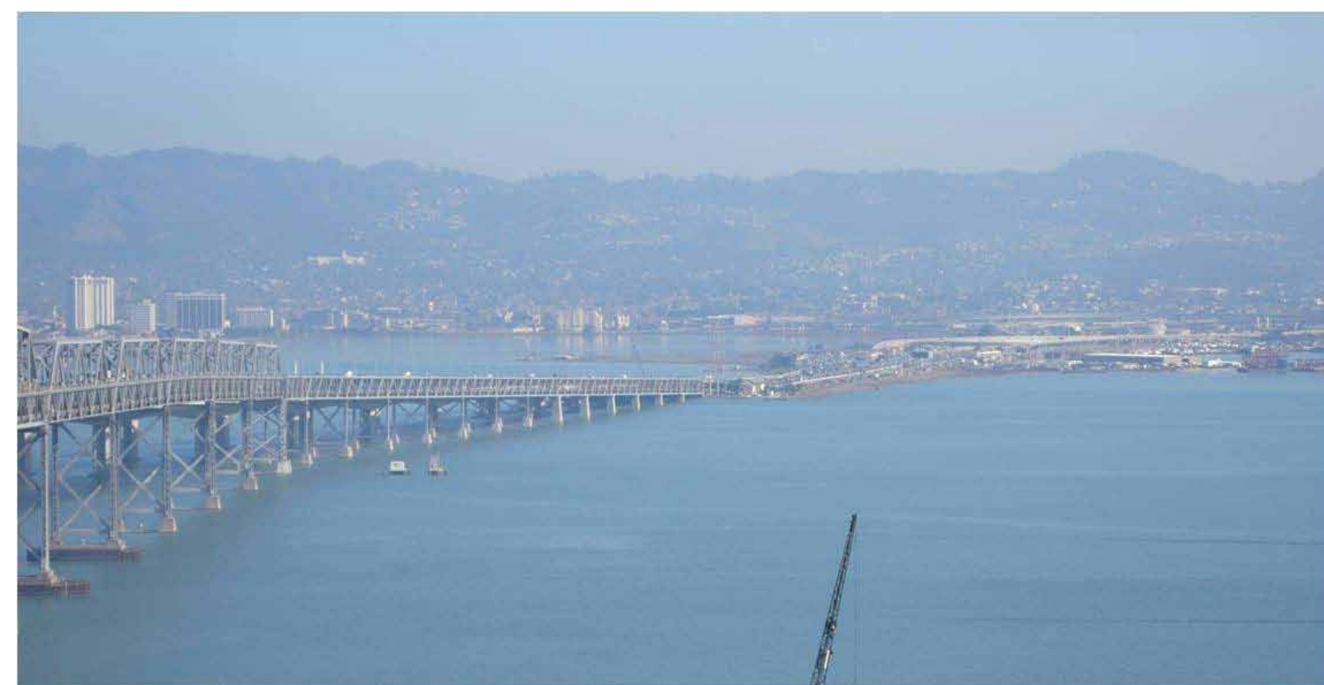
Existing East Span of Bay Bridge
