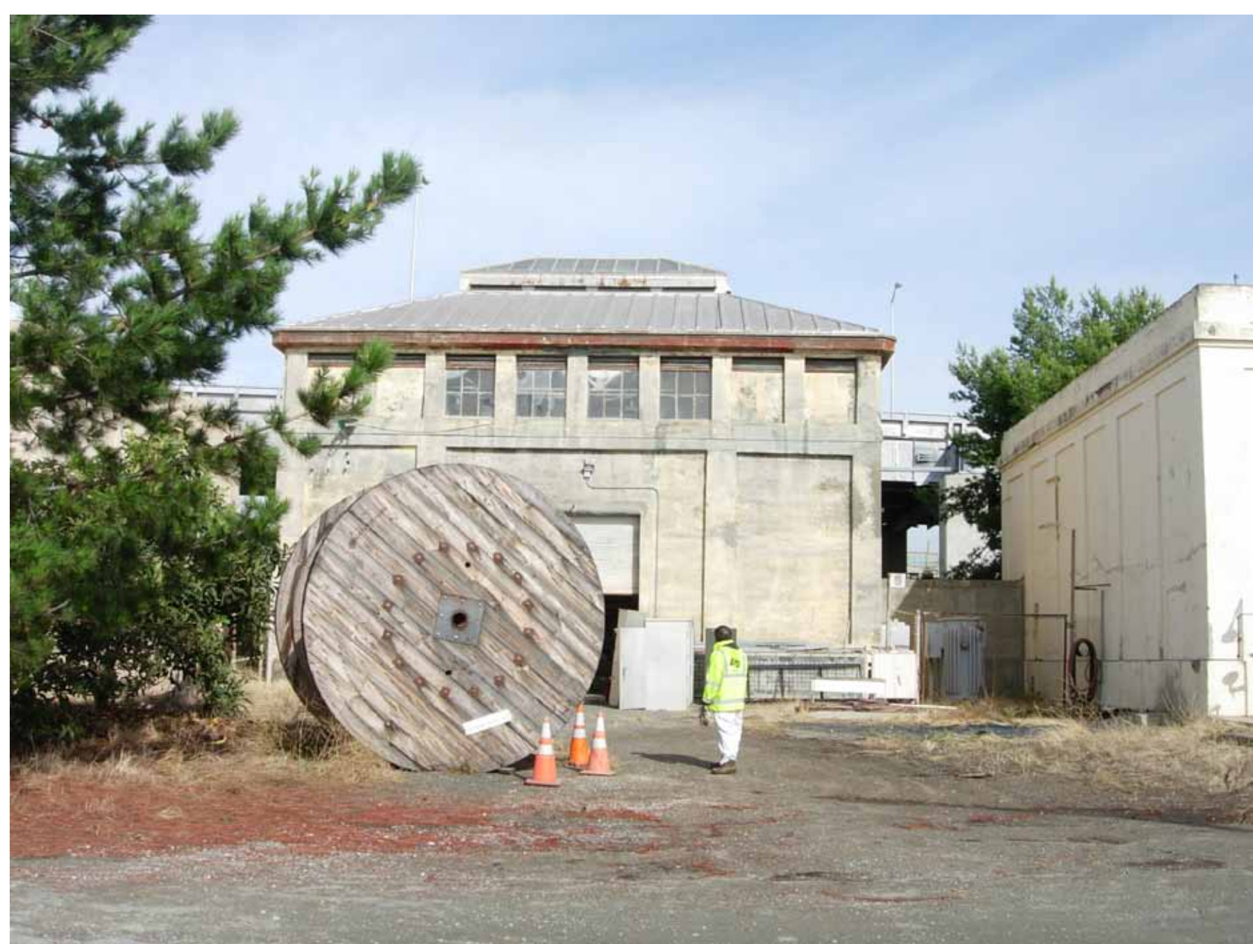
Key Pier Substation
