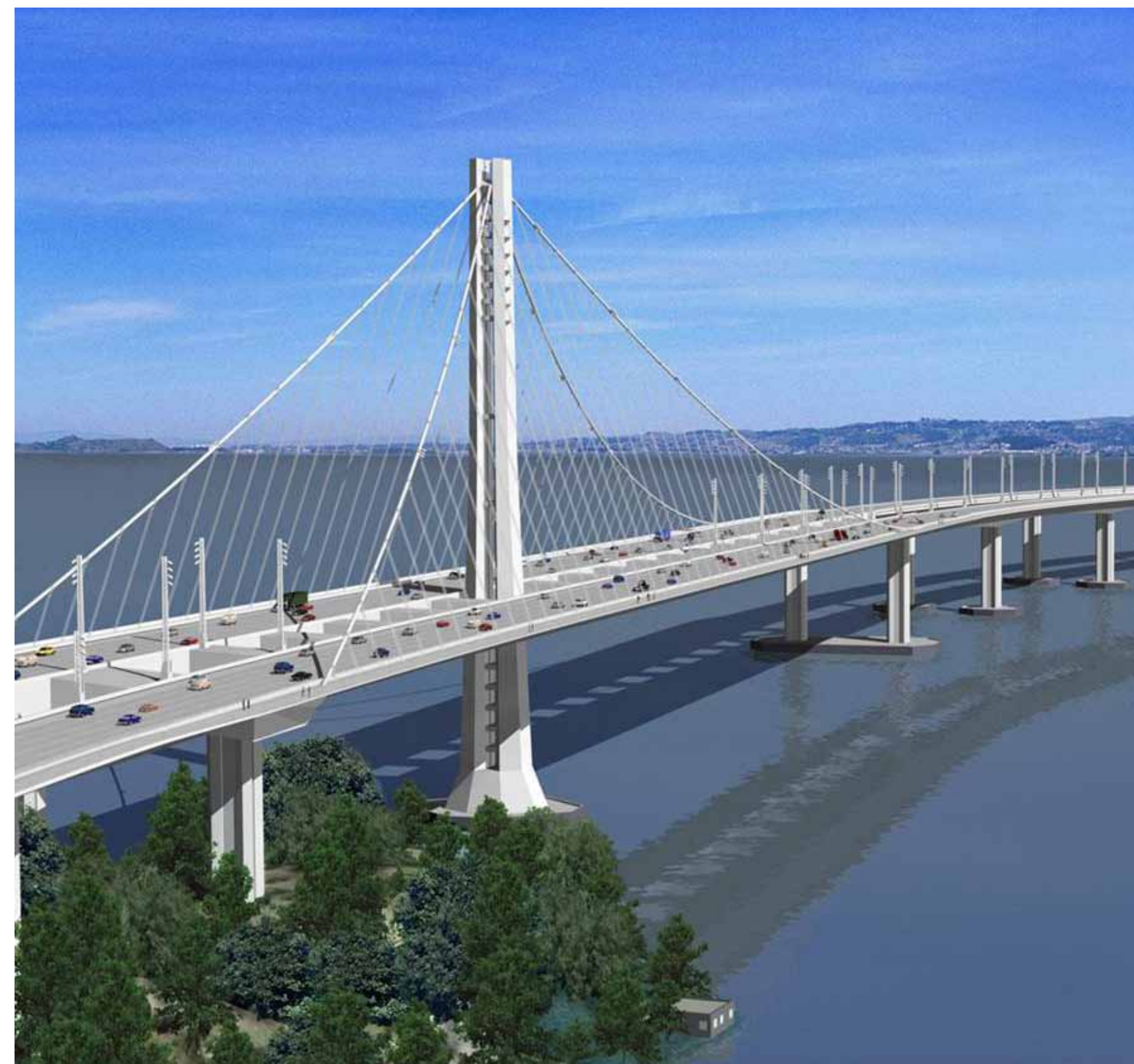
Self Anchored Suspension Bridge
