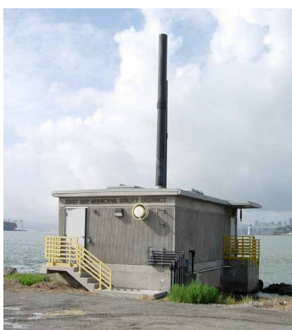
EBMUD Wastewater Treatment
